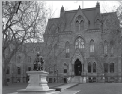
University of Pennsylvania Historic Stone Facade Repairs
